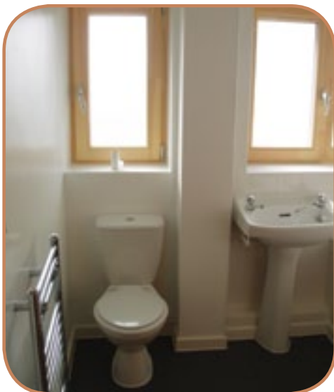
Figure 6.4 In smaller rooms, can the fixtures and fittings still be accommodated once IWI has been installed? (Source: ECD Architects)
