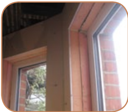
Figure 6.22 Phenolic thermal laminate boards line the inside of a bay window. (Source: ECD Architects)
