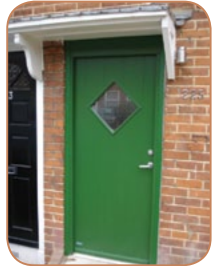
Figure 6.43 Bespoke dimensions for high performance entrance doors may not be available and make-up panels may be required above the door. (Source: ECD Architects)
