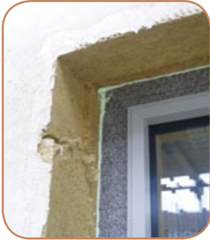
Figure 6.40 Externally insulated frames awaiting EWI to be overlapped. (Source: ECD Architects)
