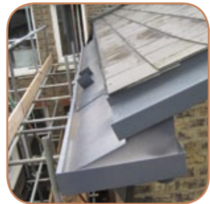
Figure 6.20 Proprietary eaves gutter and verge extensions may avoid the need to extend roof structures. (Source: Prewett Bizley Architects)
