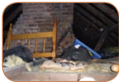
Figure 6.26 Loft spaces are often used for storage of household items and this greatly reduces their thermal performance. (Source: ECD Architects)
