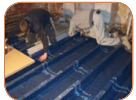
Figure 6.13 Breather membranes can be lapped tightly over and between floor joists to support loose or quilt insulation. (Source: ECD Architects)
