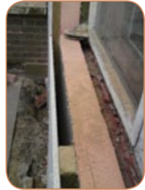
Figure 6.17 Insulated rainscreen system build-up: parge coat as air barrier; mechanically fixed insulation boards; ventilated batten zone; cement fibreboard carrier or decorative rainscreen panel. (Source: ECD Architects)
