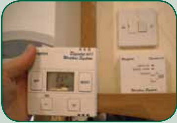
Figure 9.4.2 A wireless room thermostat.
