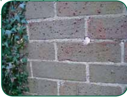
Figure 9.16 A cavity masonry wall that has been filled.
